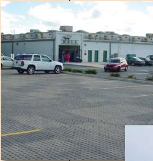
About 40,000 sf (3,716 m 2 ) of PICP eliminated the need for building detention pond when a parking lot was expanded behind a Wal-Mart shopping center.
