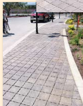
The sidewalk adjacent to the nursery entrance uses permeable paving units to return water to nearby vegetation.
