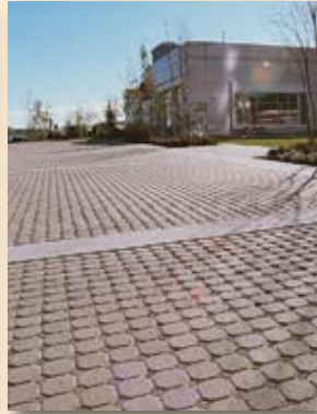
Adjacent to the Toronto SkyDome and the CN Tower in Toronto, this fire station uses PICP to reduce runoff pollutants entering nearby Lake Ontario.
