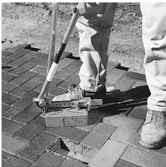
Figure 5. Using a paver extractor to remove a paver
