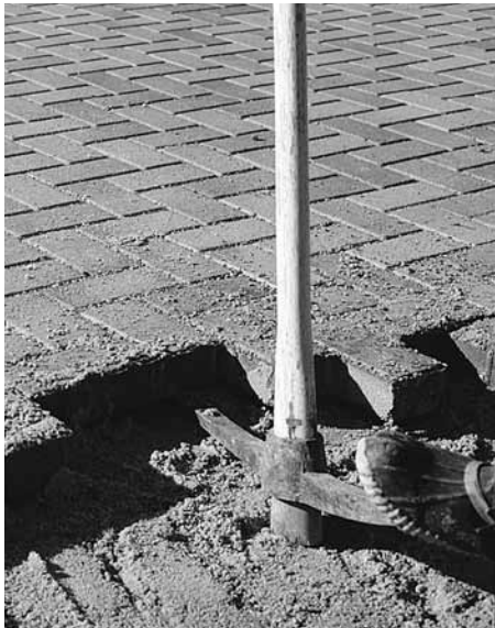
Figure 6. Prying out the remaining pavers
