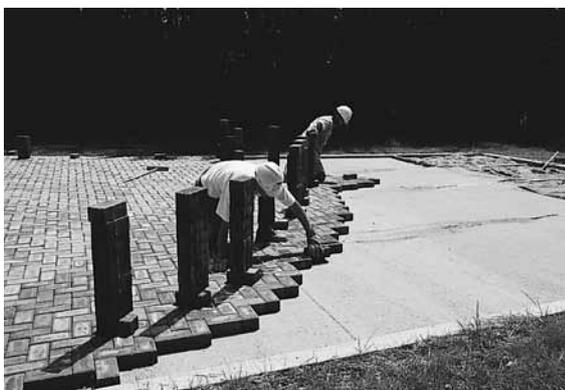
Figure 7. Placing the concrete pavers.
