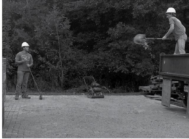
Figure 10. Spreading and sweeping joint sand.
