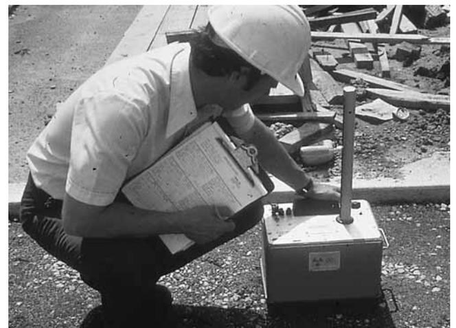
Figure 5. Density testing of the aggregate base with a nuclear density gauge.
