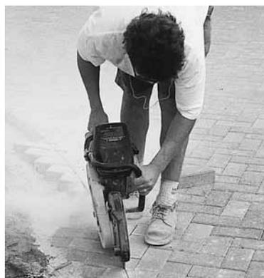
Figure 8. Saw cutting pavers.
