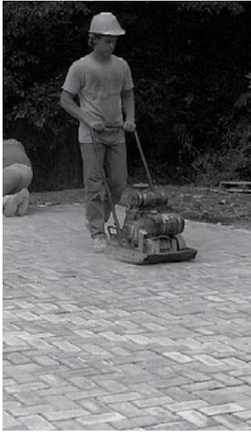
Figure 9. Compacting the pavers and bedding sand.
