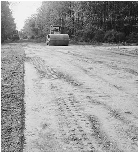
Figure 2. Compacting the soil subgrade.
