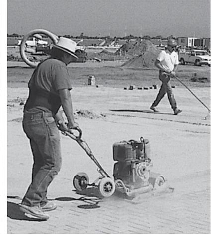
Figure 11. Vibrating sand into the joints.
