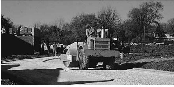
Figure 4. Base compaction with a vibratory roller.
