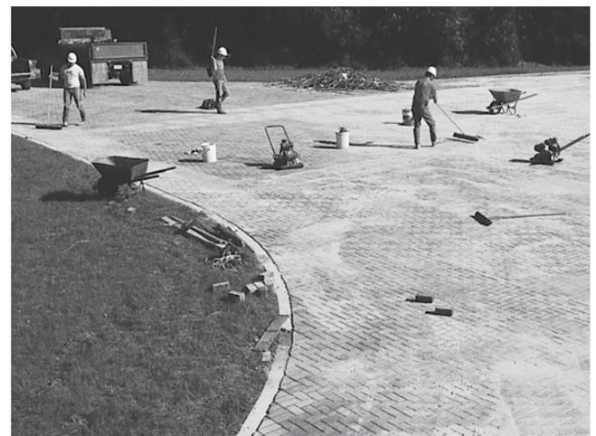
Figure 12. Excess sand swept from the finished surface will make the pavement ready for traffic.
