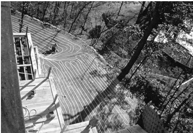
Figure 6. Experienced electrical and plumbing contractors should install snow melting systems.
