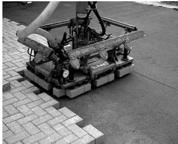
Figure 6. The vacuum head over the paver layer.
