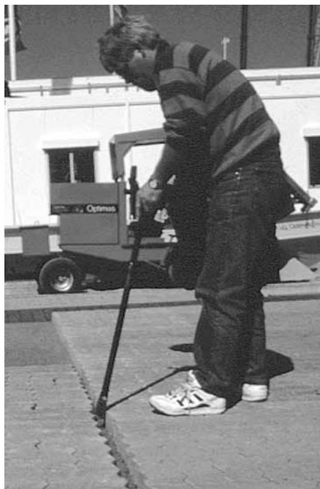
Figure 21. Once a few layers are removed by hand, then adjacent layers can be separated with a pry bar.
